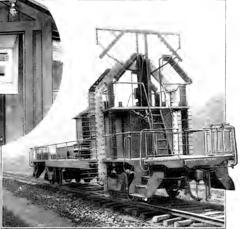
With All Attachments Working Automatically It Is Possible to Take Clearance Measurements While the Car Is Running
